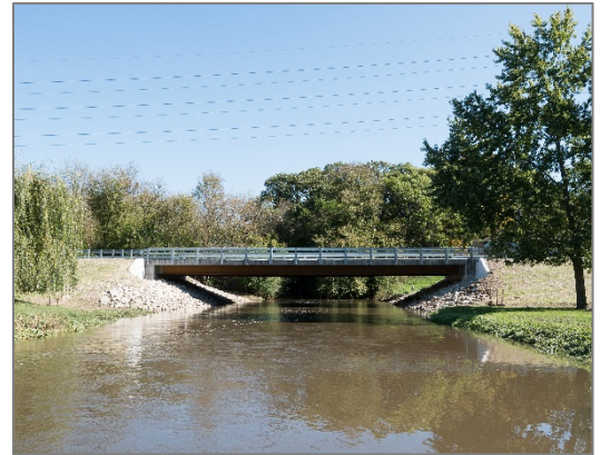
DeKalb County Highway Department Somonauk Road Bridge Replacement
